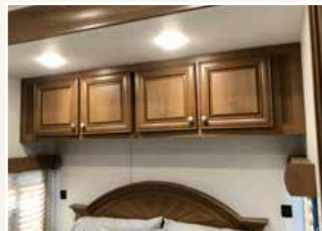
Residential Raised Panel Cabinetry.
